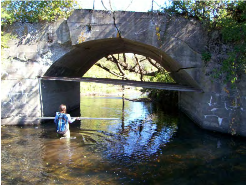
Figure 14. Farm bridge in reach R15.01-A that is structurally unsound and is causing localized geomorphic instability.
